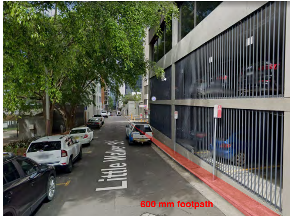
Existing Footpath Condition at No.165 (extent of pedestrian public domain shown red)
